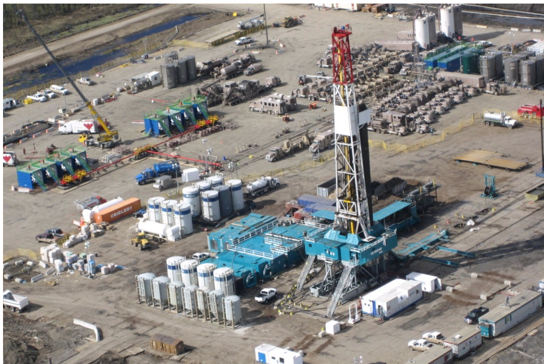
Horn River Gas Factory: 63-K Concurrent Operations May 2010
