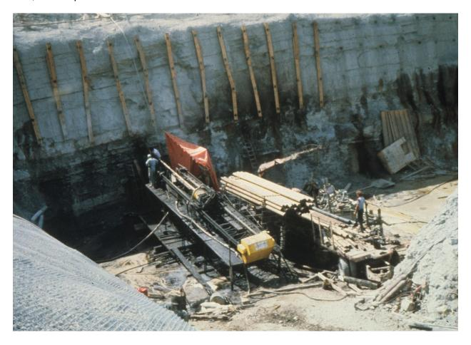
Figure 1: Hawker Siddeley Super Drill 150 in "The Pit".
