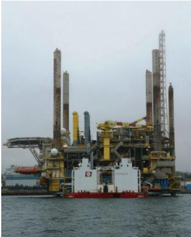
Figure 4: The decommissioned Deep Panuke field production platform in Halifax Harbour August 2020 (Photo credit Kristie McVicar).
