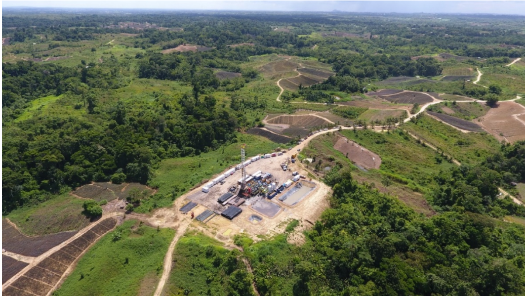
Fig 4: Drone footage of the COHO-1 Exploration Wellsite
