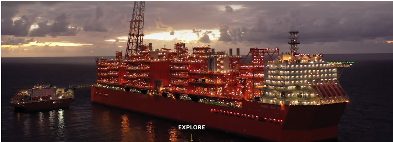
Figure 8. ENI operated Coral South FLNG facility. From ENI website, March 2, 2024
