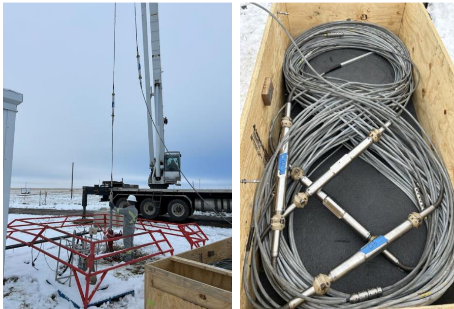
Figure 1 the picture on the left shows the deployment of the downhole array and the picture on the right shows a close up of the tools with the FO wireline cable separating each receiver station by 15 meters.
